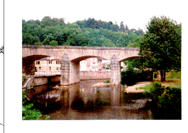
Pont de la RD127 (Cousin-le-Pont) Sbv = 348,79 km 2 P10 = 62 mm/jour Q10 = 65 m 3 /s Q100 = 130 m 3 /s
